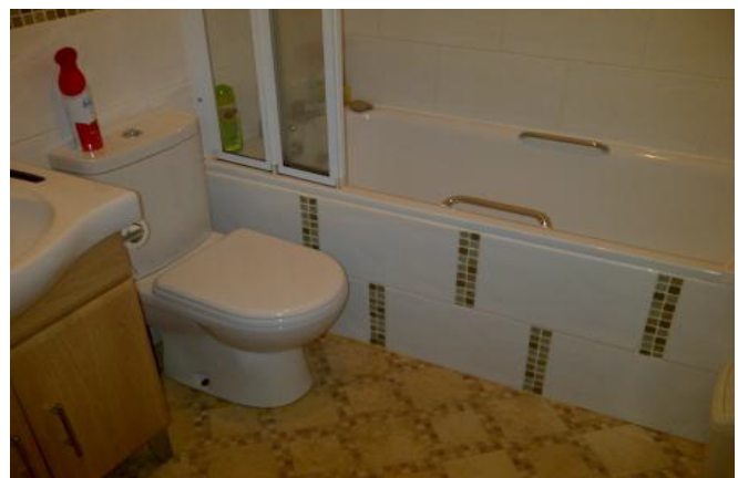
▶ Typical bathroom and WC
